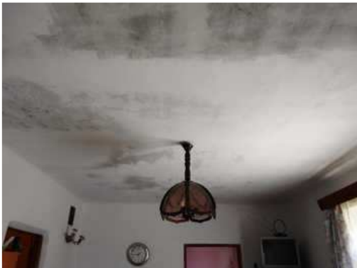
strop v kuchyni
